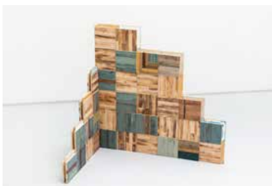
Figure 64 > Indoor wall made from used interior wood
