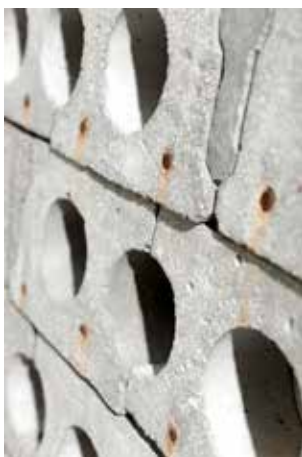
— Figure 75 Concrete bricks made from concrete slabs
