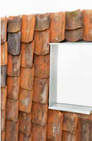
— Figure 77 Facade cladding made from roof tiles
