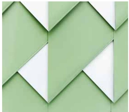
- Figure 48-51 Steel roofing sheets turned into facade shingles- Right image of surface painted shingles
