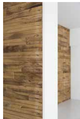
- Figure 9 / Dismantled floorboards from renovation repurposed as wall cladding, Vandkunsten in Albertslund Syd, 2014.
