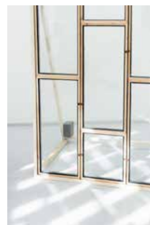
— Figure 73 Glass facade made from used glazed windows
