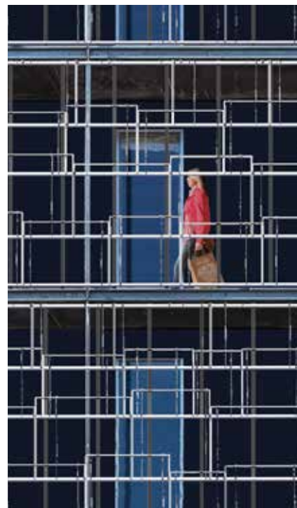
- Figure 32-34 Illustration of facade system with preused windows and wires.
