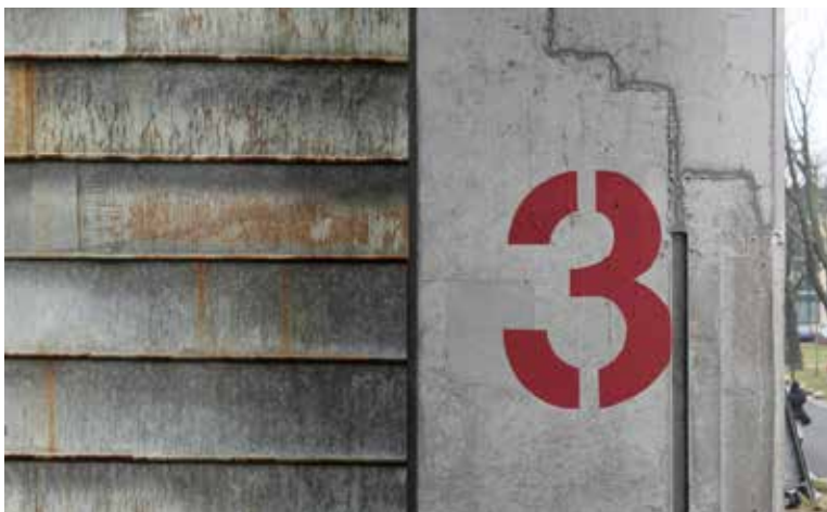
- Figure 48-51 Steel roofing sheets turned into facade shingles- Right image of surface painted shingles
