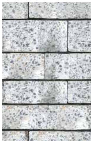
Facade from cut concrete blocks.
