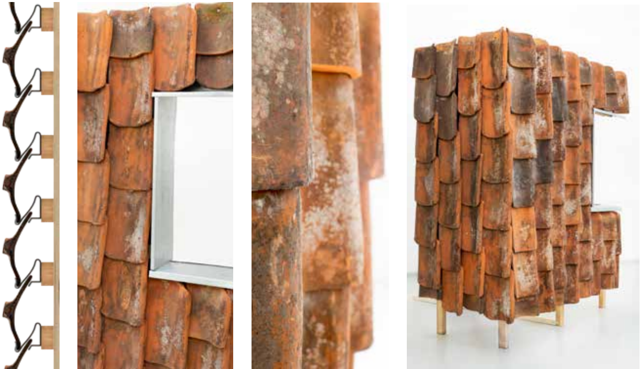
- Figure 16 left / section of system with backside out. Fig 18-19 / Details of prototype of pantile facade system
