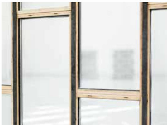
Figure 63 > Glass facade made from used glazed windows
